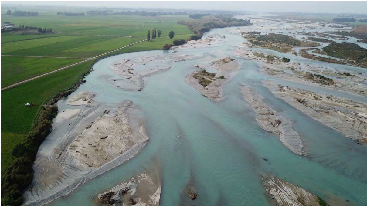
Drone photograph showing bank erosion at Tawai farm – note the heavily vegetated islands, pushing the flow of water towards the banks.
