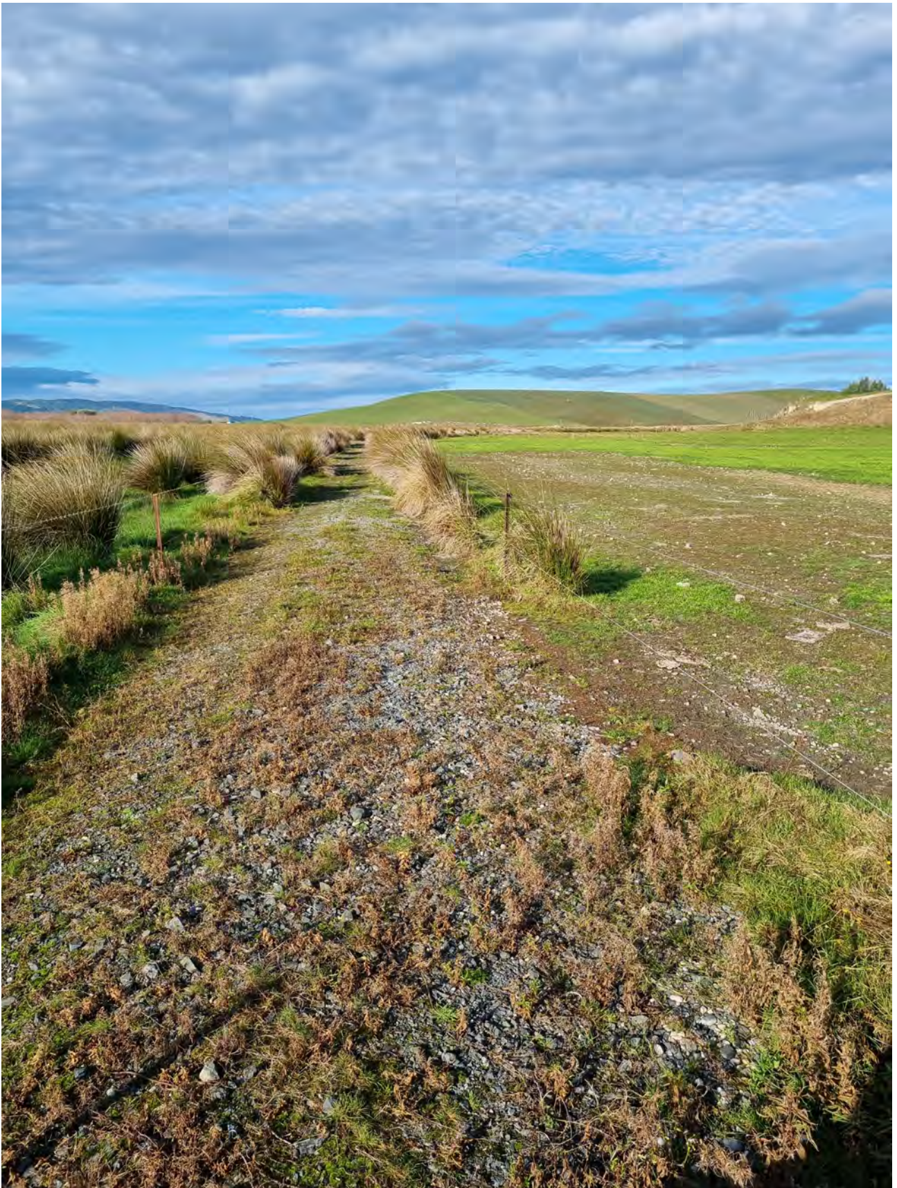
Illustration 1: Figure 2: Although dry in dry summers, regular ponding and flooding causes grass to die and track to be inaccessible without gumboot. Photo taken on 7 May 2021
