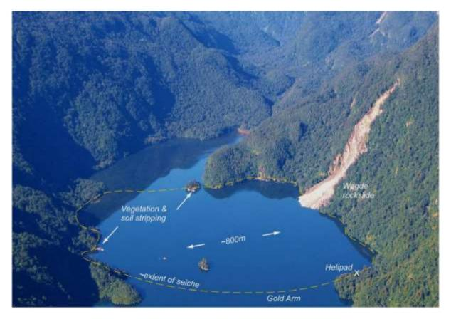
Figure 9. The 2003 Fiordland earthquake caused a 200,000 m<sup>3</sup> rockslide into Charles Sound. The landslide caused a small tsunami, which ran 4-5 m up the other side of the sound, approximately 800 m away (*Hancox et al.*, 2003).
