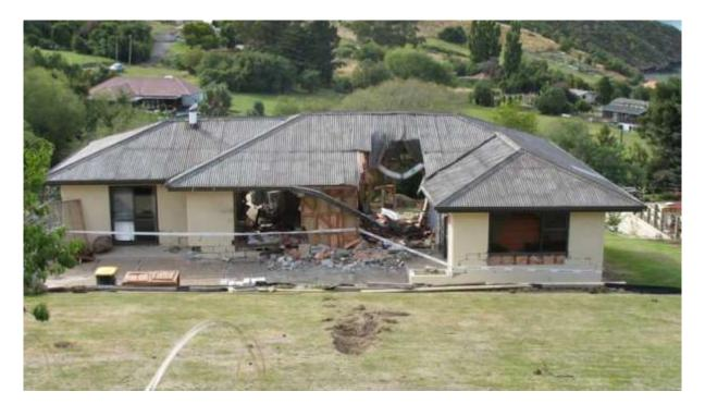
Figure 8. Rockfall damage to dwelling at Rapaki, Christchurch, during Feb. 22nd 2011 earthquake. The gouge in the foreground is an impact divot from a boulder, which then impacted the house (photo courtesy D. Barrell, GNS Science).
