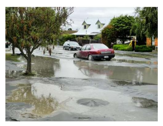
Figure 6. Liquefaction in Avonside following the February 21 Christchurch 2011 earthquake (photo by Martin Luff, Wikipedia Commons).
