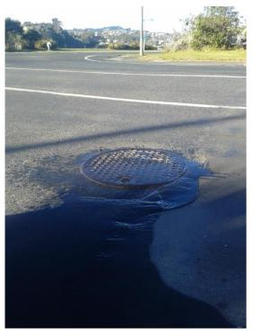
Figure 39. Sea water rising up through the stormwater system on Teviot Street at about high tide, 2:30pm on 6 May 2016. The pressure in the stormwater pipe below this man-hole cover is such that it has pushed water up above ground level. This was not the highest tide experienced during that month. Photograph source, ORC.
